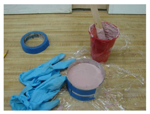
12. Remove the tape around the form allowing the form to unroll. Remove the form. The plaster is very weak at this point. Handle it with care.
